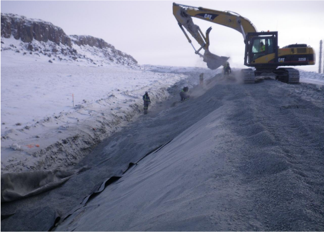
Photo 6: Diversion Berm – HDPE liner under the uncompactd crush slid down the slope.
