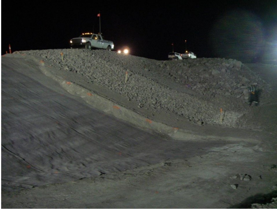
Photo 10: North Dam – preparations for placement of overliner core material. Note the grade marks on the crest of the previously placed overliner material. Photo looking north from Sta. 0+40.
