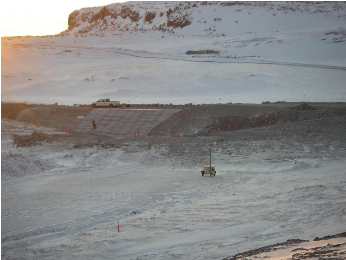
Photo 9: North Dam – General view of the North Dam. Note extent of the GCL liner placed on dayshift. Photo looking west.
