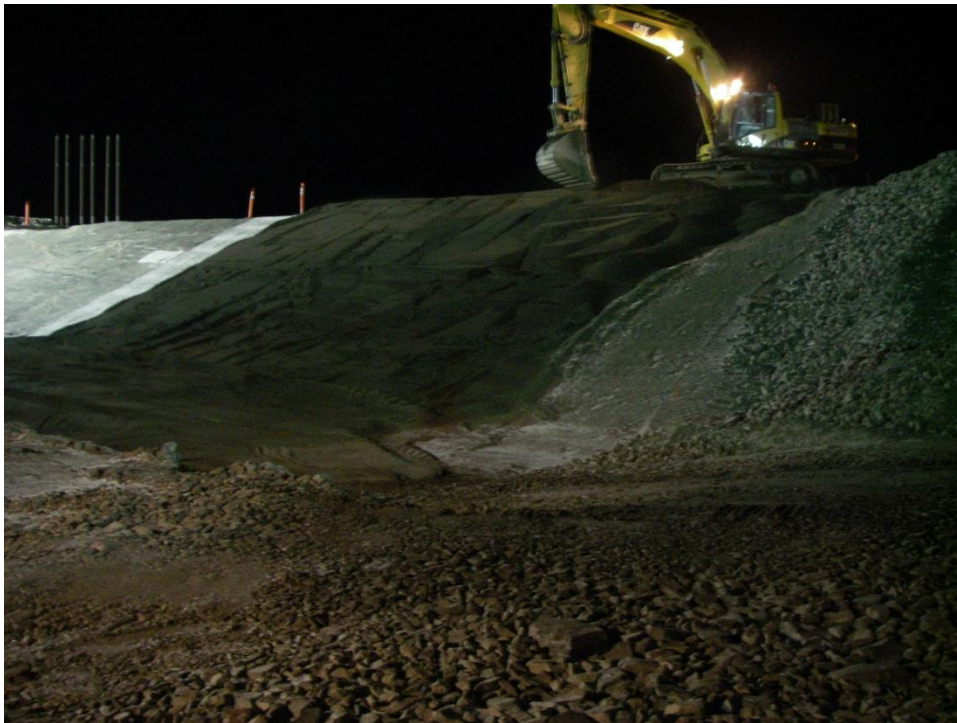
Photo 11: North Dam – finishing the surface of the placed overliner core material, before compaction. Photo looking south-west, from Sta. 0+90.
