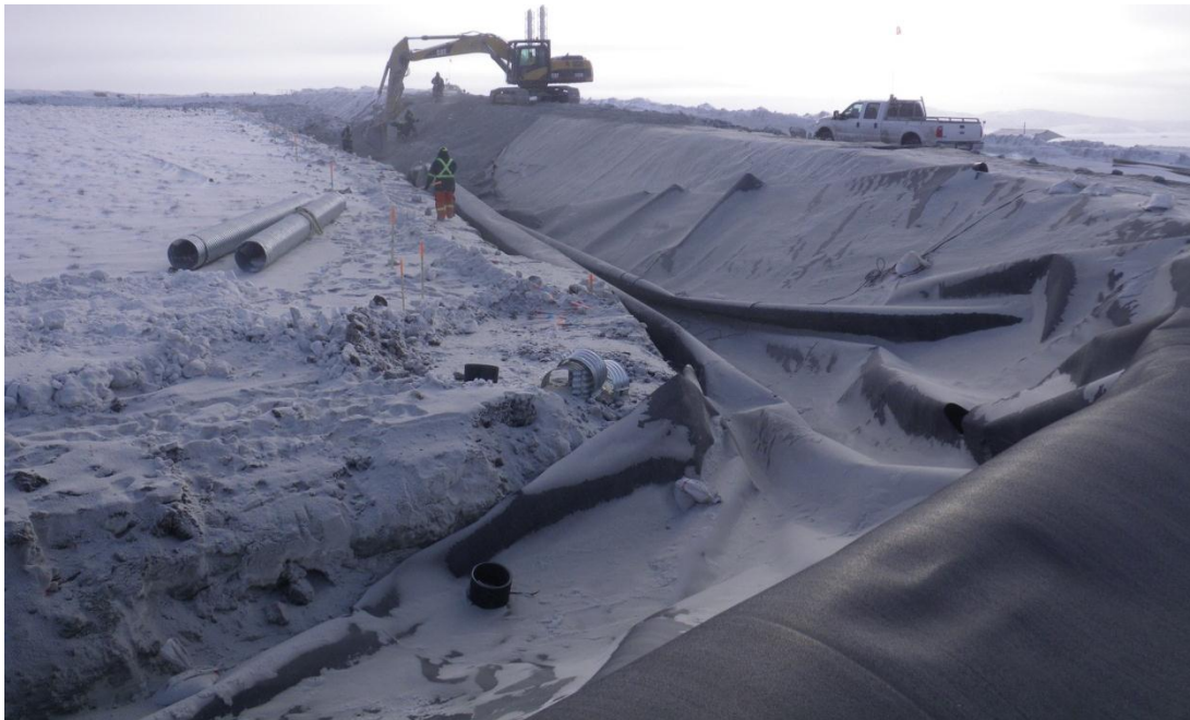
Photo 5: Diversion Berm - Liner and geotextile slid down the slope at the diversion berm near the culvert crossing. Photo looking south east.
