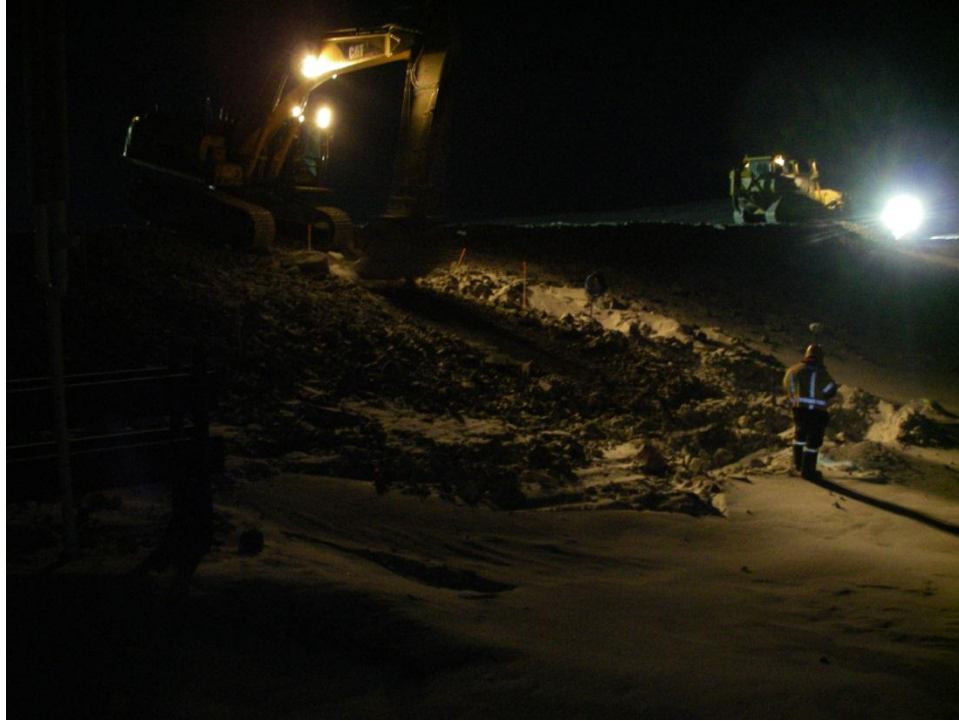
Photo 14: North Dam – finishing the downstream slope of the dam around Sta. 1+75. Surveyor is providing grade control support to the excavator operator. Photo looking south from the ice road.
