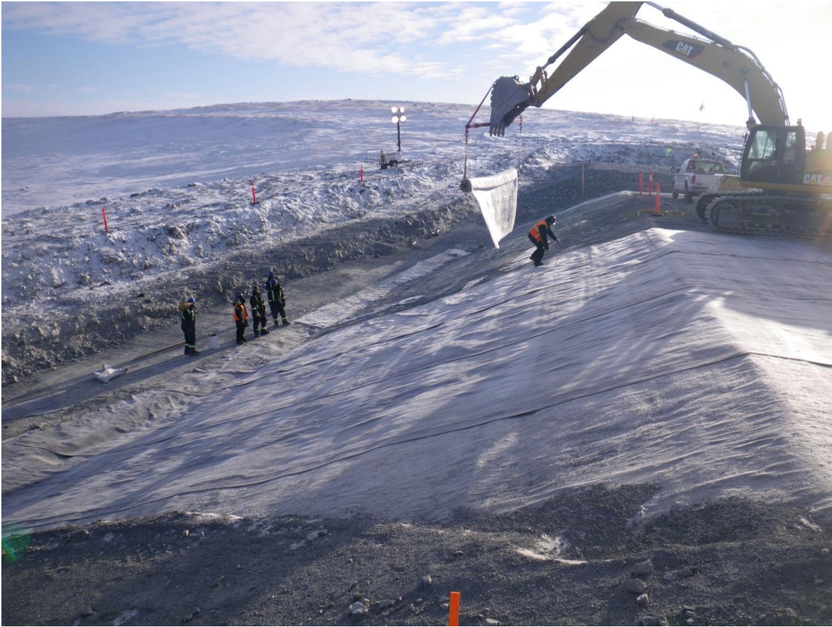
Photo 4: North Dam – GCL being placed along slope.
