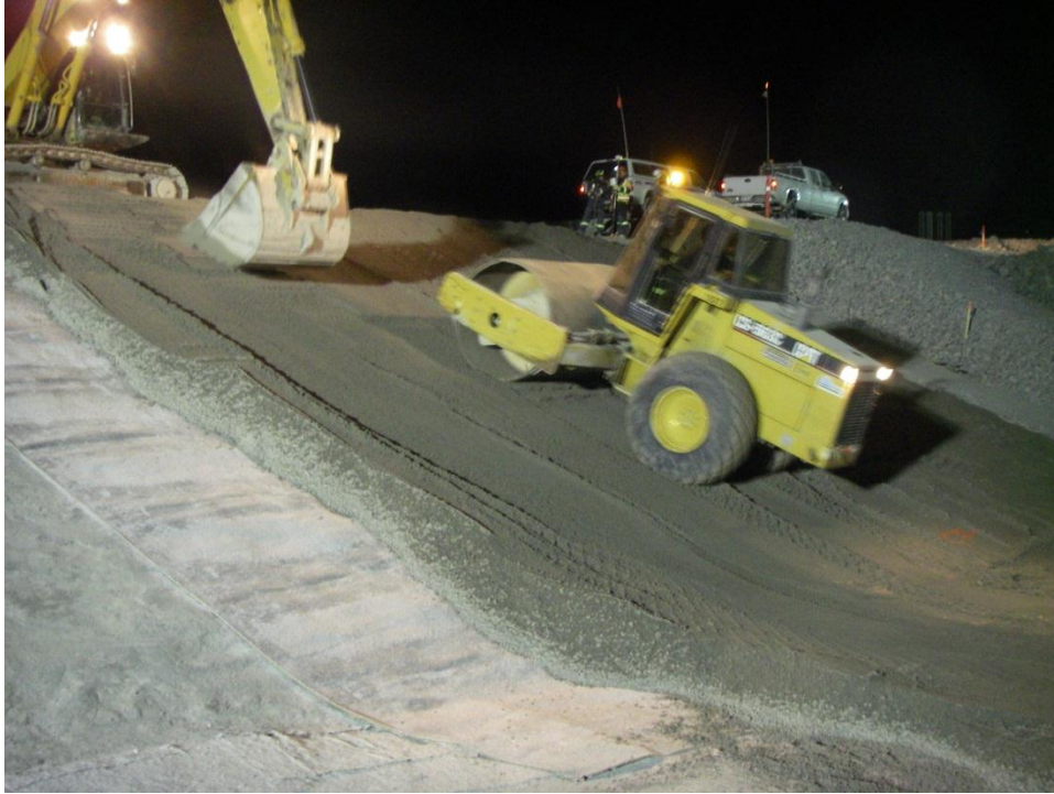
Photo 12: North Dam – compacting the placed overliner core material. Photo looking north from Sta. 0+50
